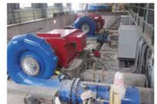
Asiga River small hydroelectric plant - Water turbine generators
