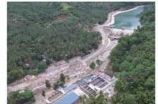
Water supply project (water intake facility)
